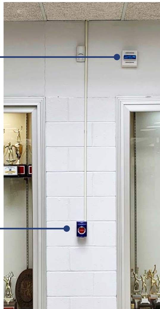
Lockdown Panic button & notification strobe installed throughout the building.
