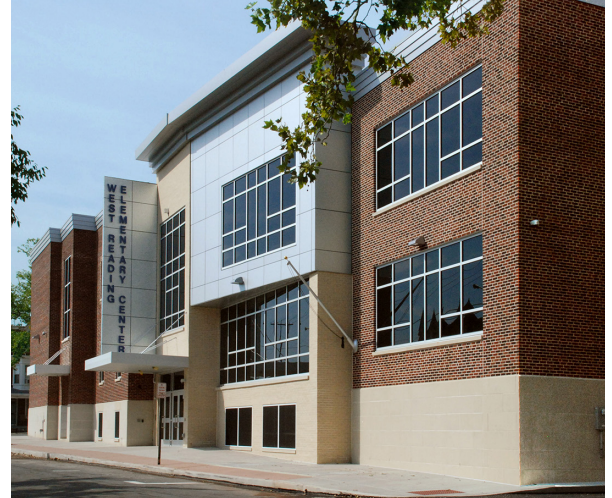
West Reading Elementary Center
