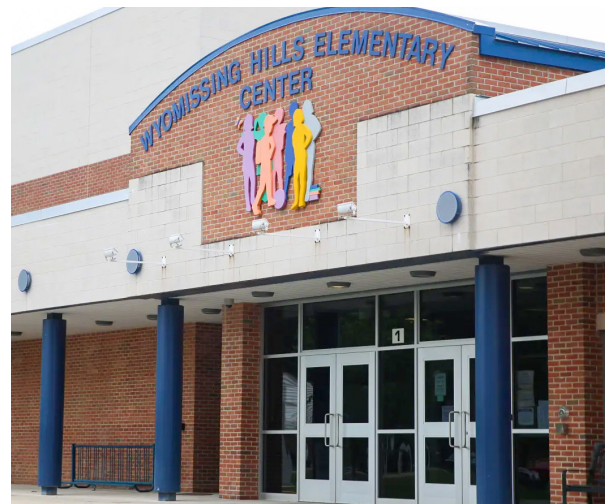
Wyomissing Hills Elementary Center
