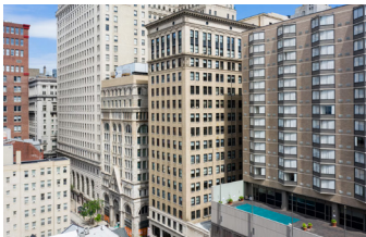
The Philadelphia Building 1315 Walnut St.
