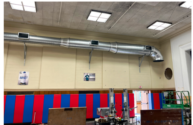
Ductwork installation process
