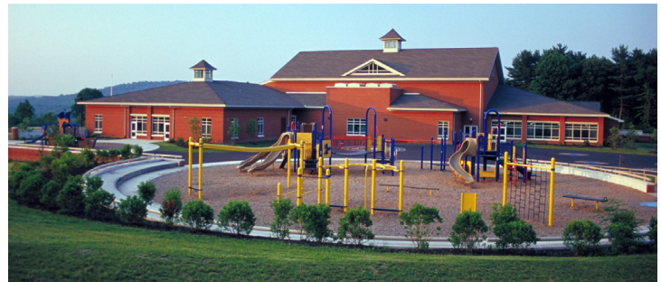
Schwenksville Elementary School
