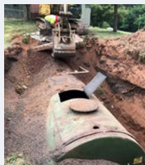
Oil Tank Relocation
