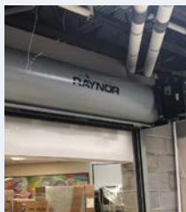
Relocated, Modified Overhead Door
