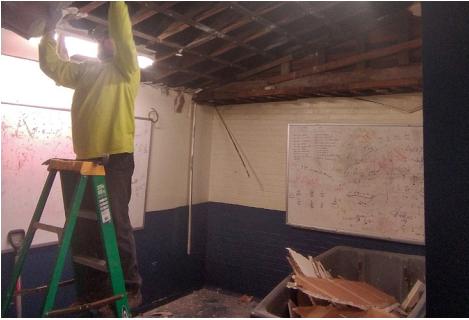
Demolition phase of lead remediation program
