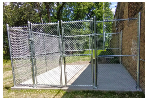
Concrete pad with fence for new HVAC unit, moved from interior to exterior to maximize space
