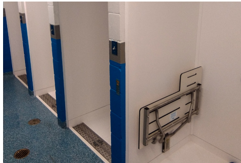
New showers with easy-clean structure and privacy features
