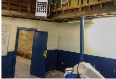
Demolition continues with complete material removal
