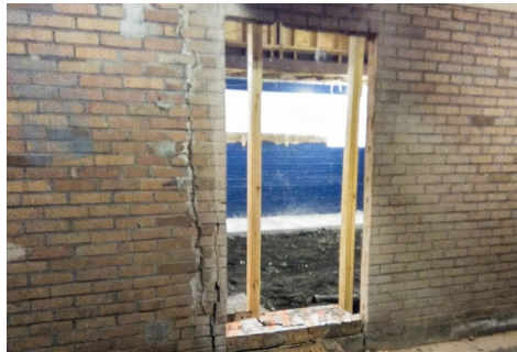
A second mode of egress was added in accordance with ADA requirements
