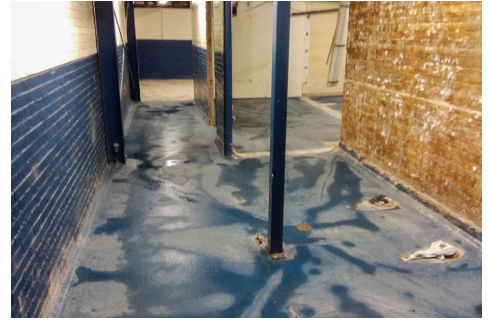
Beginning of epoxy floor process
