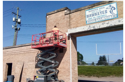
Brick repointing to welcome stadium visitors and showcase the newly renovated stadium and field house
