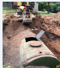
Oil Tank Relocation
