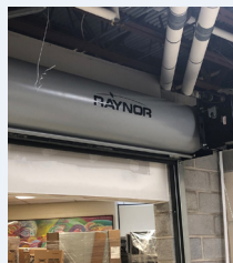
Relocated, Modified Overhead Door
